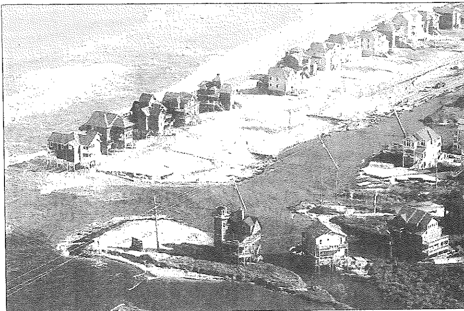
A road is flooded Sunday in Hatteras Island, N.C., after Hurricane Irene swept through the area Saturday.
