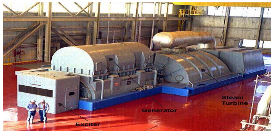
Figure 7: Three-phase power generator (Electric Power Research Institute)
